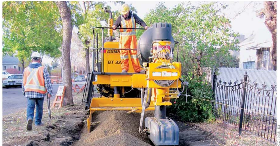
An aggregate base mold prepares the grade and features a spreader auger. The aggregate material is placed in front of the machine and the auger spreads the material the width of the mold. The trailing pan features three pan vibrators for the initial compaction of the base material.
