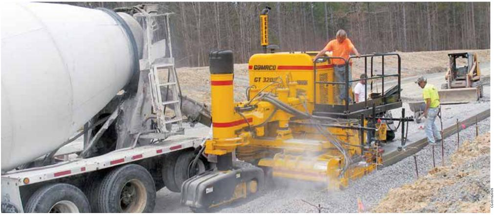
GOMACO's GT-3200 features the simultaneous trim/pour concept for maximum concrete utilization. The trimmerhead has 36 inches (914 mm) of sideshifting and 14 inches (356 mm) of hydraulic vertical lift adjustment capabilities.
