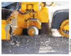
The trimmerhead has ample power to trim crushed gravel base.
