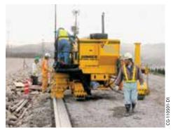
The GT-3200 can be controlled with 3D stringless machine guidance.
