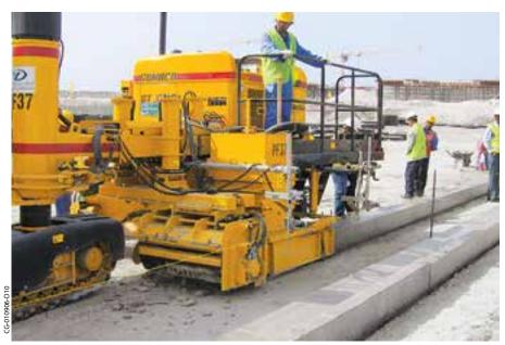
The GT-3200 features a 5.8 foot (1.77 m) long GOMACO-designed charging auger for concrete delivery to the hopper.
