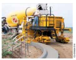
The GT-3200 slipforms curb and gutter around a radius on a subdivision project.
