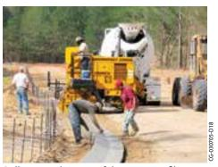
Roll-over curb is one of the many profiles a GT-3200 can slipform.
