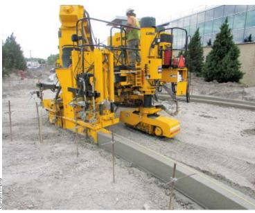
The operator's platform on the Xtreme GT-3600 is isolated to reduce vibration for a comfortable day of paving curb and gutter.
