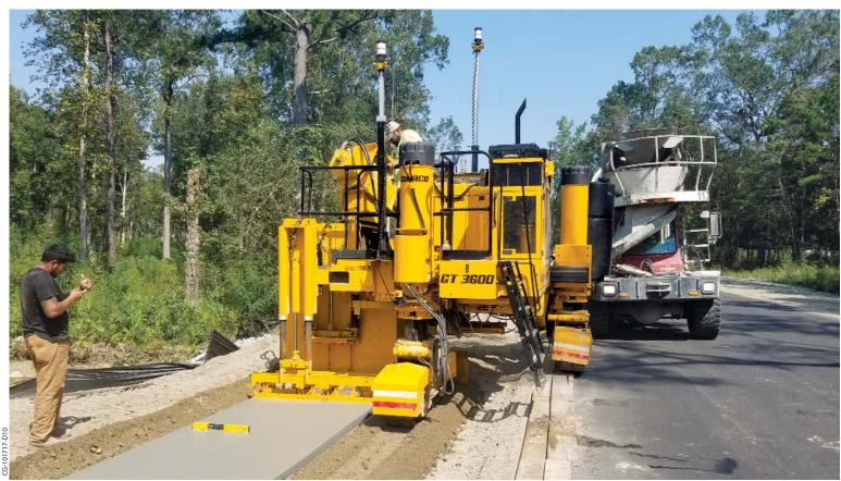
The GOMACO Xtreme GT-3600 slipforms a five foot (1.52 m) sidewalk with 3D machine guidance.
