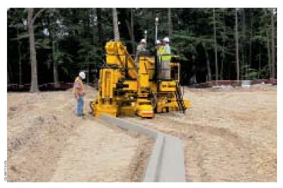
The Xtreme GT-3600 slipforms curb and gutter in a developing area using 3D machine guidance. The intelligent All-Track Positioning on the Xtreme GT-3600 includes a smart hydraulic cylinder on all three legs. The smart cylinders allow G+® to know the position of all three tracks and can make steering adjustments as needed.
