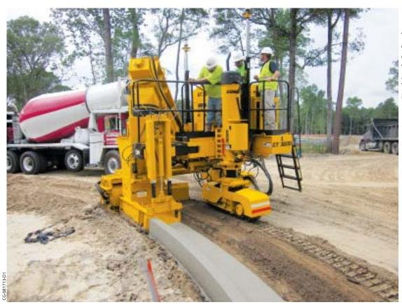
The Xtreme GT-3600 slipforms curb and gutter with 3D machine guidance. The extreme steering capabilities, combined with the Xtreme GT-3600's sensored All-Track Steering and sensored All-Track Positioning, make it the ultimate, intelligent slipform paver.
