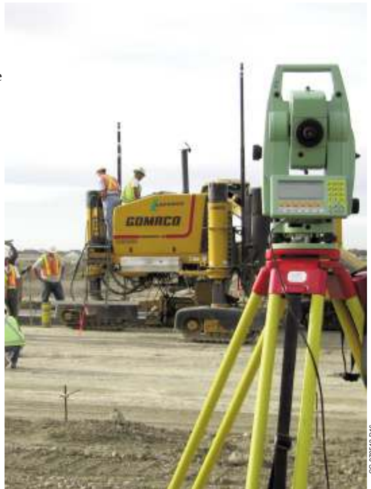
A Commander III uses 3D stringless control to slipform curb and gutter.
