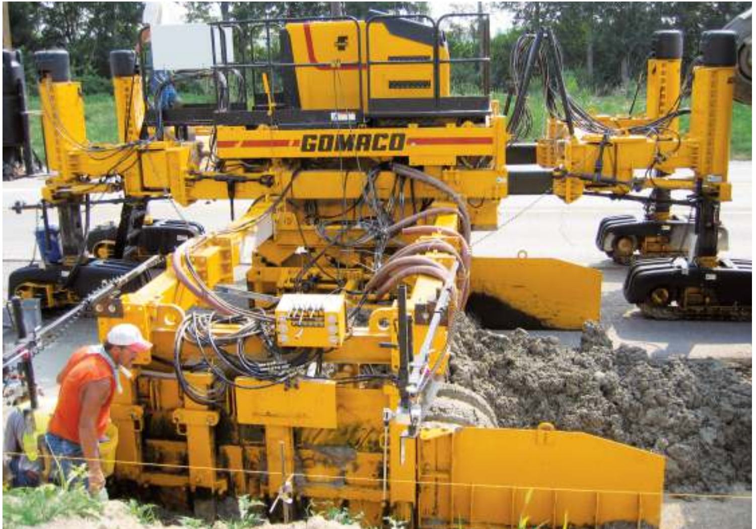
A Commander III four-track with an 11 ft. 6 in. (3.51 m) wide sidemounted mold slipforms a new shoulder with integral curb while operating in Reverse Steer to pave with the traffic flow.
