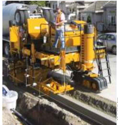
This Commander III provides high-production slipforming curb and gutter below grade on a city street in Canada.
