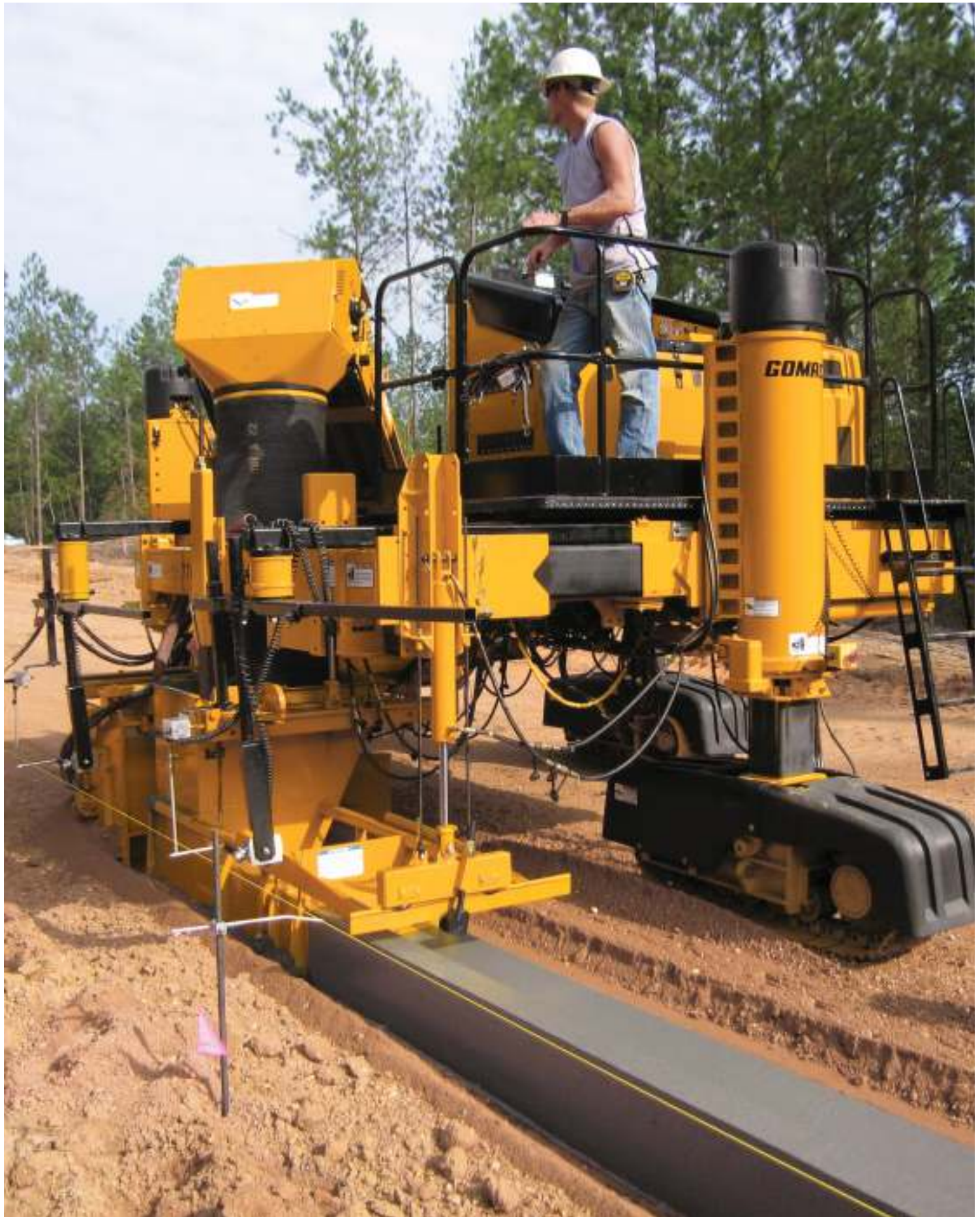
A Commander III three-track simultaneously trims through 2.5 inches (64 mm) of Mississippi red clay as it slipforms 24 inch (610 mm) wide stand-up curb and gutter on a new housing development.
