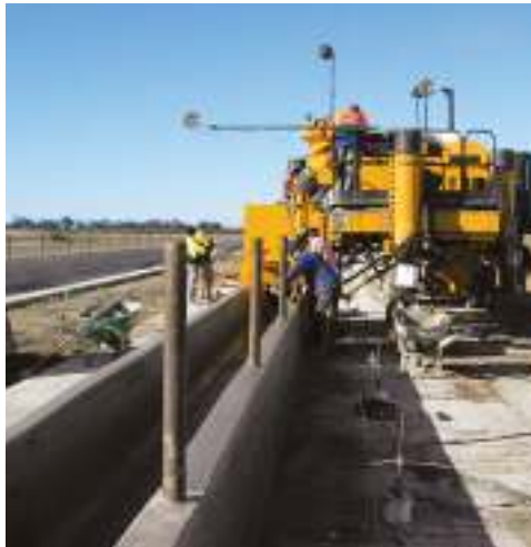
The feed bunk mold has a hydraulic pipe inserter mechanism that allows the insertion of 4 ft. 3 in. (1.3 m) long pipes into the sidewall of the new feed bunk on-the-go while slipforming.
