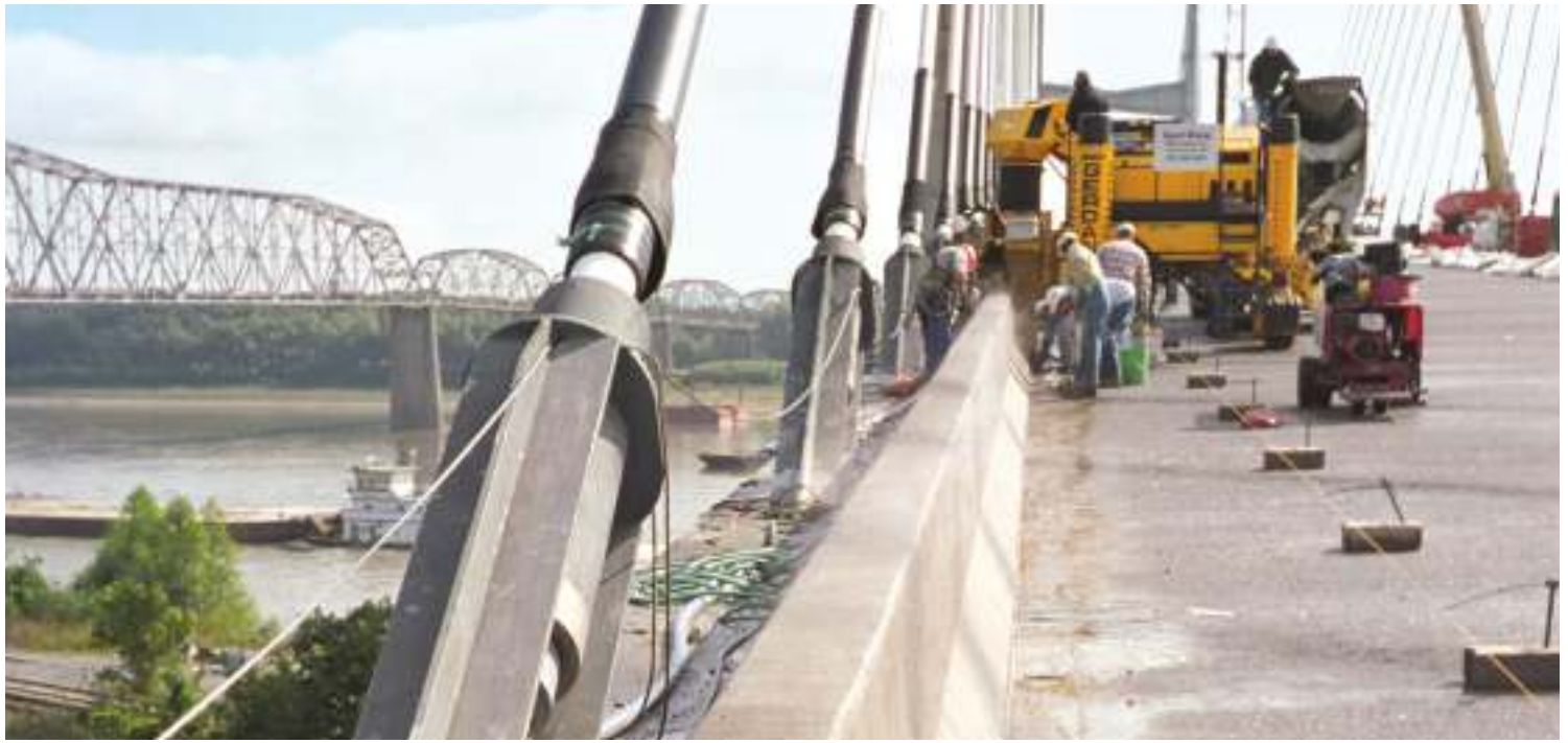
A Commander III three-track slipformed 14,500 ft. (4420 m) of three different types of barrier and parapet wall on this project in Missouri. The parapet above measures 18 in. (457 mm) wide at the top, 36 in. (914 mm) at the base and 34 in. (864 mm) tall.
