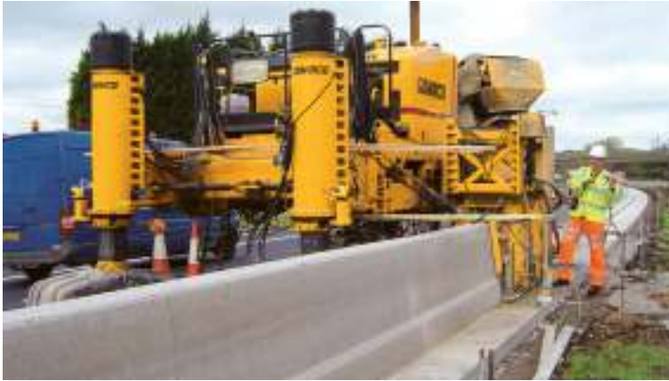
A contractor in England slipforms right-side step barrier. The exclusive digital control system allows for multiple applications and configurations, which gives the Commander III its exceptional versatility.
