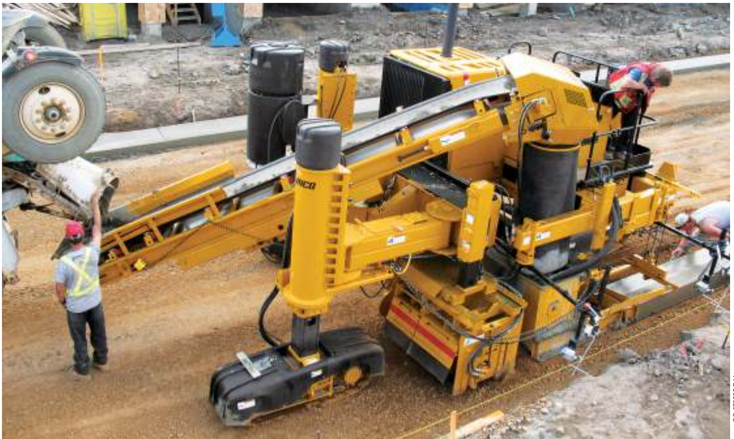
A Commander III three-track slipforms roll-over curb and gutter on a new housing development. The development featured some challenging tight working conditions and several 16 ft. 5 in. (5 m) radii.
