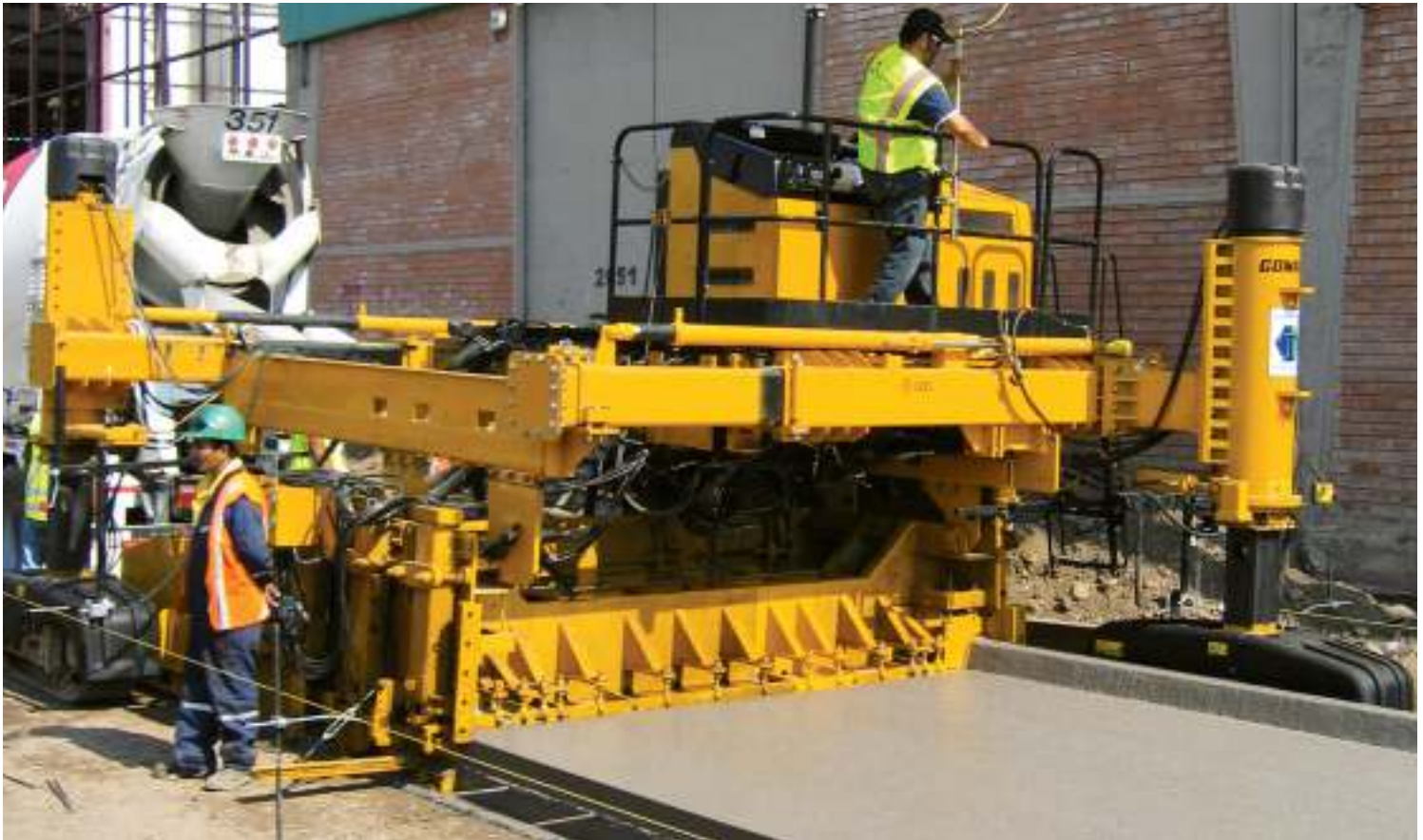
This Commander III with the 12 ft. (3.66 m) paving package attachment is slipforming a street with integral curb on one side and a side-mounted bar inserter on the other. The new roadway is being paved half-width, 11 ft. 6 in. (3.5 m) wide.
