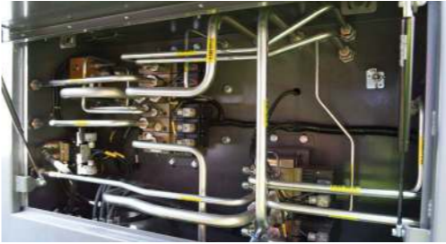
Steel pipework for better heat dissipation
